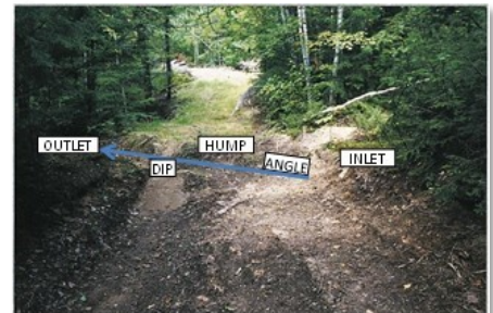
Parts of a typical water bar.
