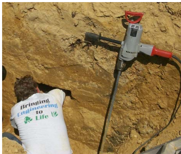
Figure 4. Holes were excavated through the sides of the trenches to place lysimeters.
