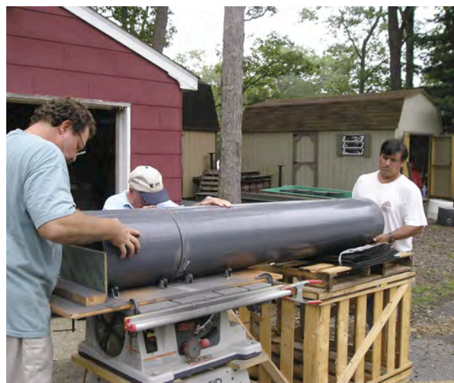
Figure 4. Keeping the pipe supported and level while cutting is very important.
