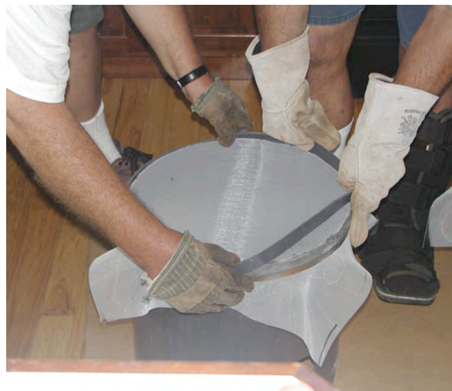
Figure 16. Stretch the warmed ring onto the glued area of the silo and allow it to set up and dry.
